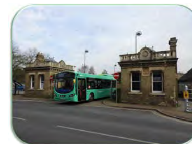
St Ives bus station
